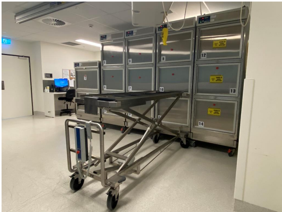
From left to right: 2 berth bariatric mortuary fridge, 4 banks of 3 berth standard mortuary fridge, bariatric cadaver stretcher lifter. Picture taken at Northern Beaches Hospital, NSW Australia.
