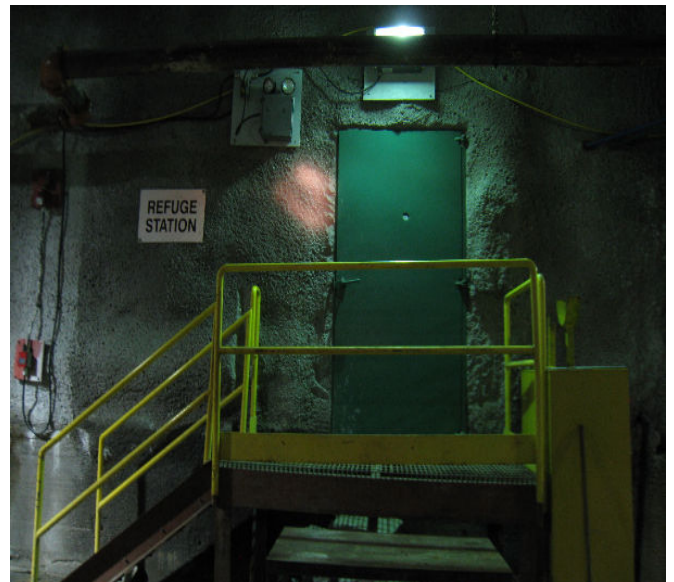
FIGURE 7 REFUGE STATION AIRLOCK
